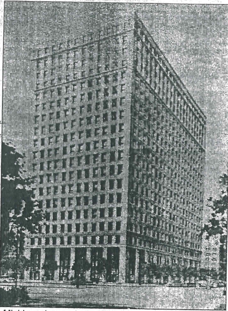
Michigan Avenue Lofts, 910 S. Michigan Ave., was built in 1911 as a furniture store. Its designers also designed the Drake Hotel in Chicago.
